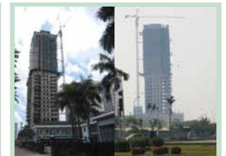
CT Licogi 13 Tower
